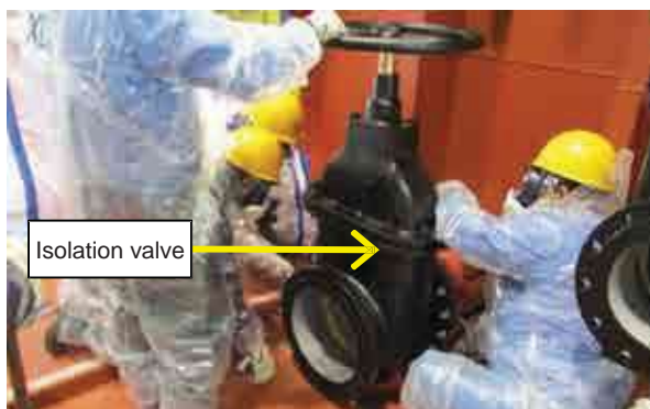
(e) Isolation Valve bolt fastening
