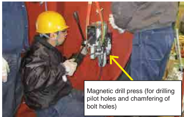
a) Bolt hole cutting
