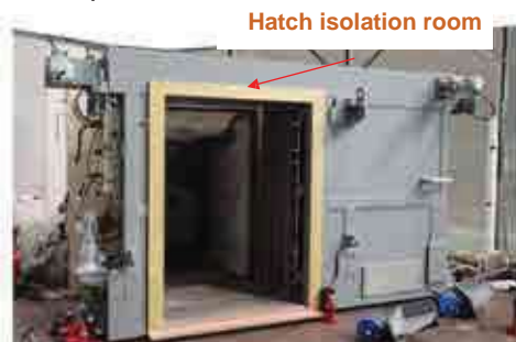
After in-stage isolation room and hatch isolation room are connected
